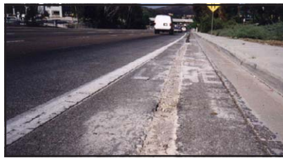
Trench right down the middle— thing of the past?
